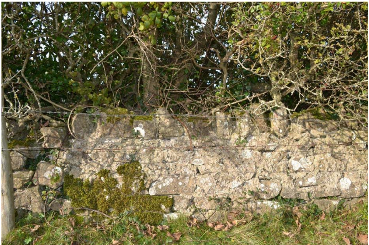
Plate 18: Detail of drystone wall construction (Gaz. 19)
